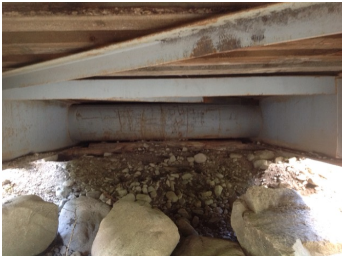
left bank bearing
