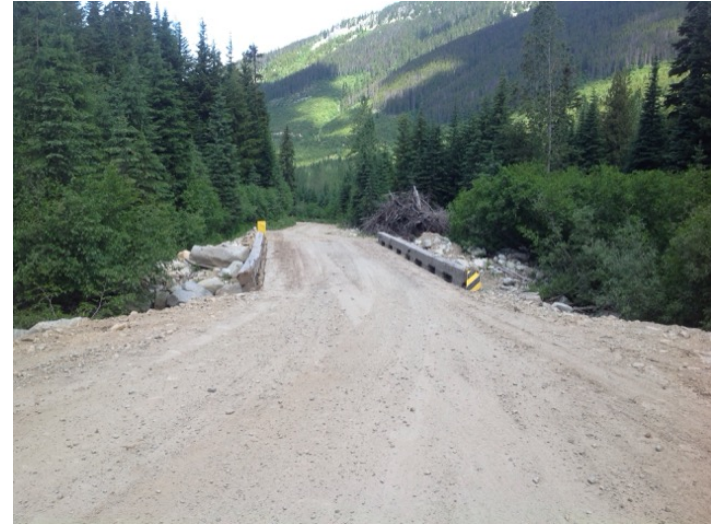
Approach from Right Bank when facing downstream
