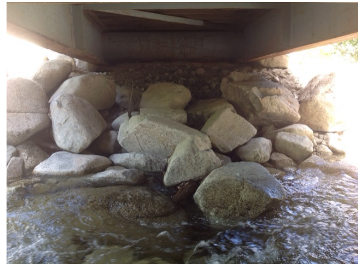
Left Bank Abutment when facing downstream
