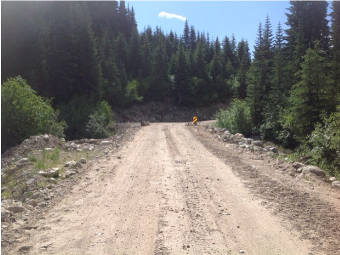
Approach from Left Bank when facing downstream
